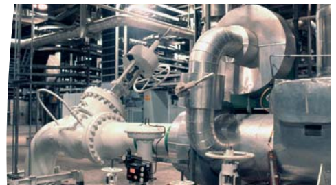
Oil refineries, offshore oil platforms, control rooms, circulating pumps for fluids, radio systems.
